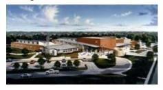
The McKinney Sustainable Elementary School Project incorporates many environmentally friendly design principles, including rainwater collection, daylighting, wind energy, solar energy, geothermal heating and cooling, and the use of recycled building materials. The Raleigh, North Carolina–based Innovative Design and EBN's Nadav Malin were environmental consultants on this project.
